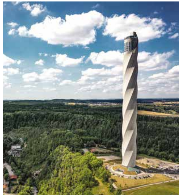
TK Elevator Test Tower Rottweil, Germany
