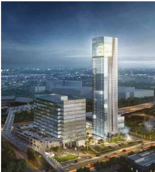
TK Elevator Test Tower Atlanta, U.S.
