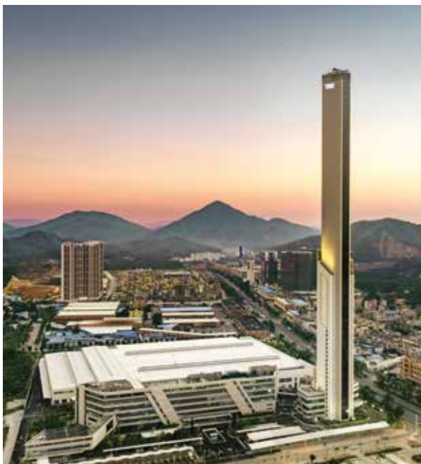
TK Elevator Test Tower Zhongshan, China
