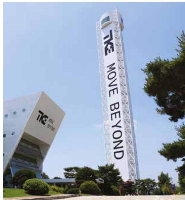
TK Elevator Test Tower Cheonan, South Korea
